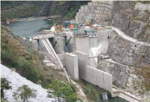
720 MW Mangdechhu HEP, Bhutan (INR 5012.63 Crores )
