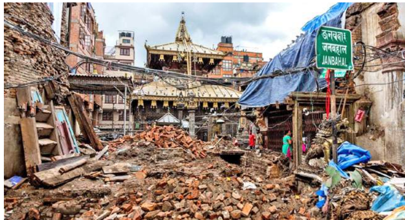
| Seto Machindranath Temple and surroundings just after the 2015 earthquake. PHOTO CREDIT: shutterstock
